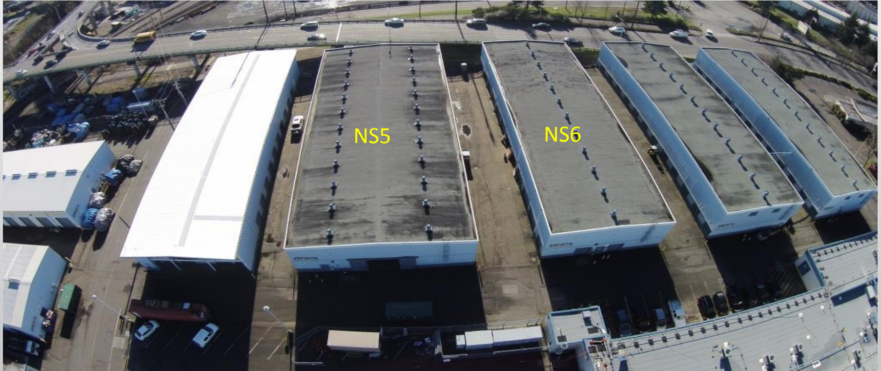
Existing Roof – Looking South
