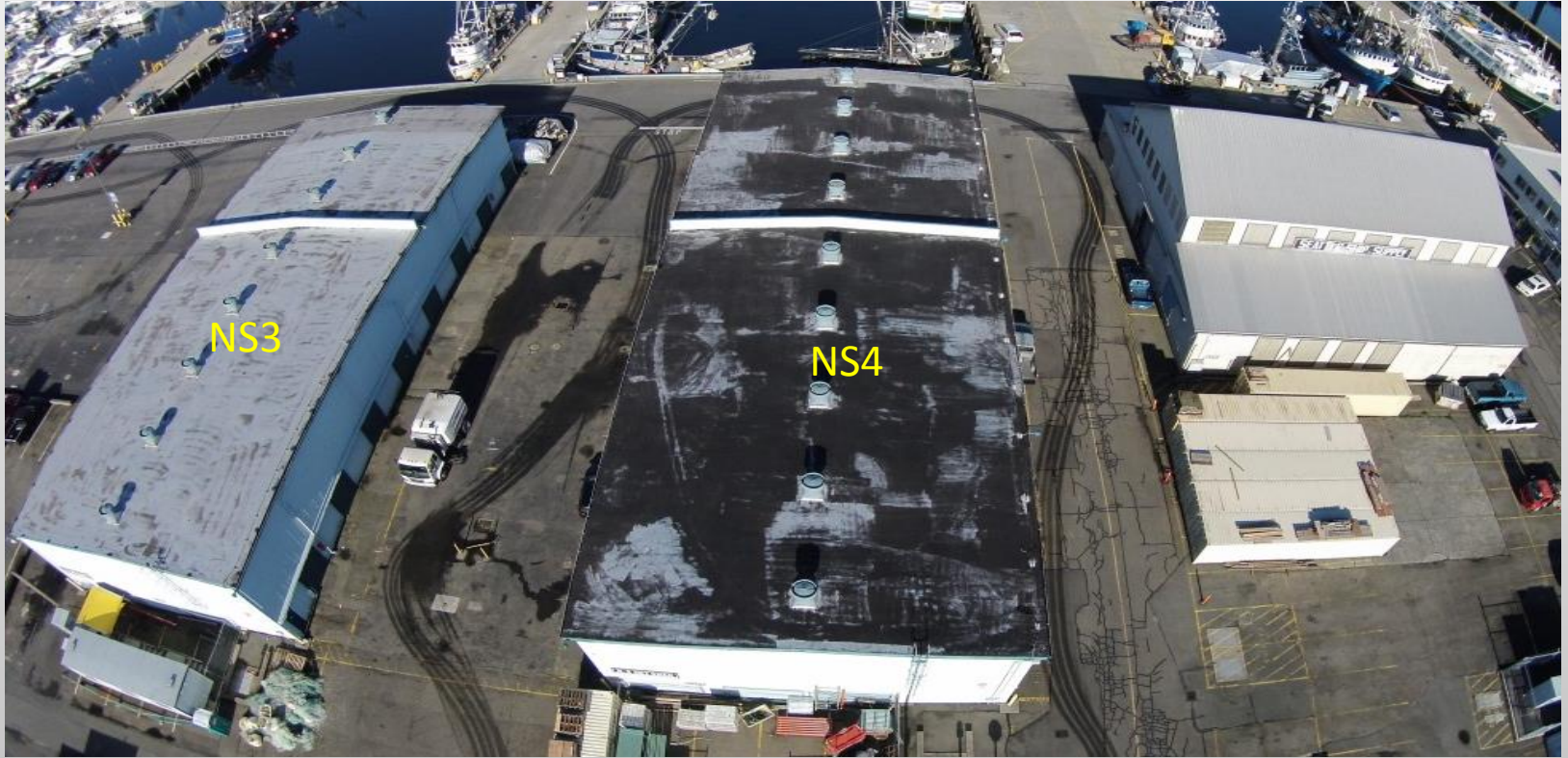
Existing Roof – Looking North
